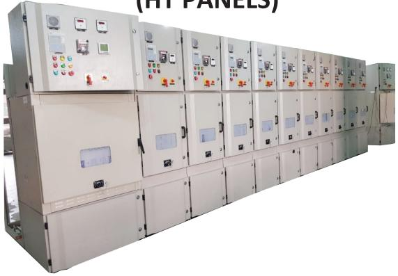
A VCB Panel is a types of circuit breaker where the arc quenching occurs is vacuum environment. VCB technology is ideal for medium voltage application .vacuum circuit breaker is renowned technology for medium voltage today and is also know as the most reliable current interruption technology for medium voltage switchgear.
